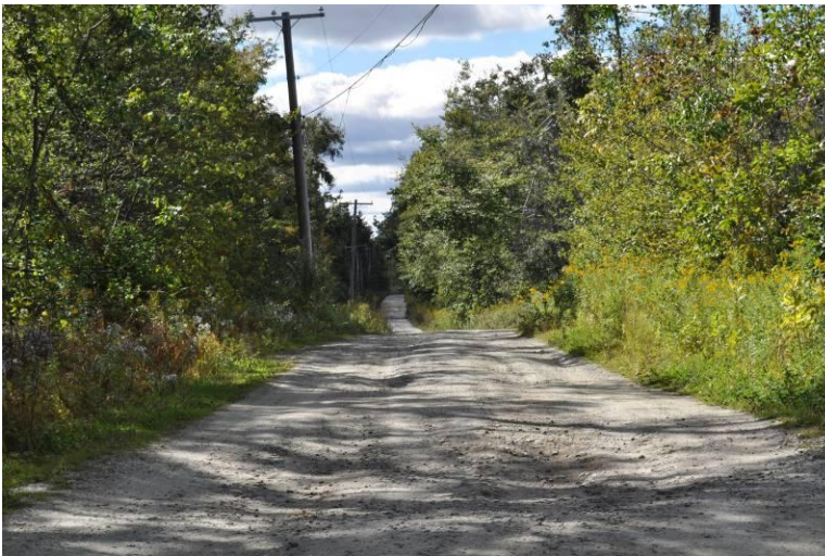
Figure 4 – Typical Conditions for Existing Pole on Unpaved Roadway
