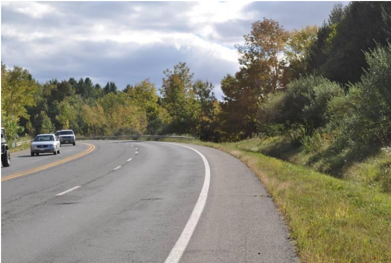
Figure 3 – Typical Conditions for New Pole Installation
