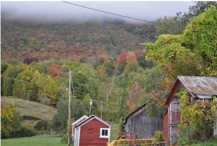
Figure 6- Existing Pole Line to Mount Greylock
